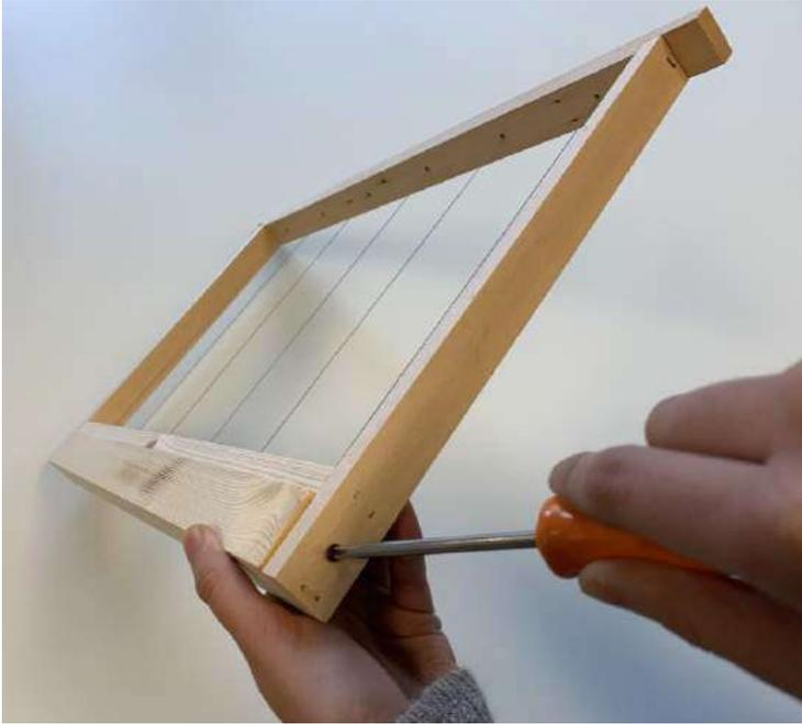
1. Unscrew the screws on the outside of the frame.
